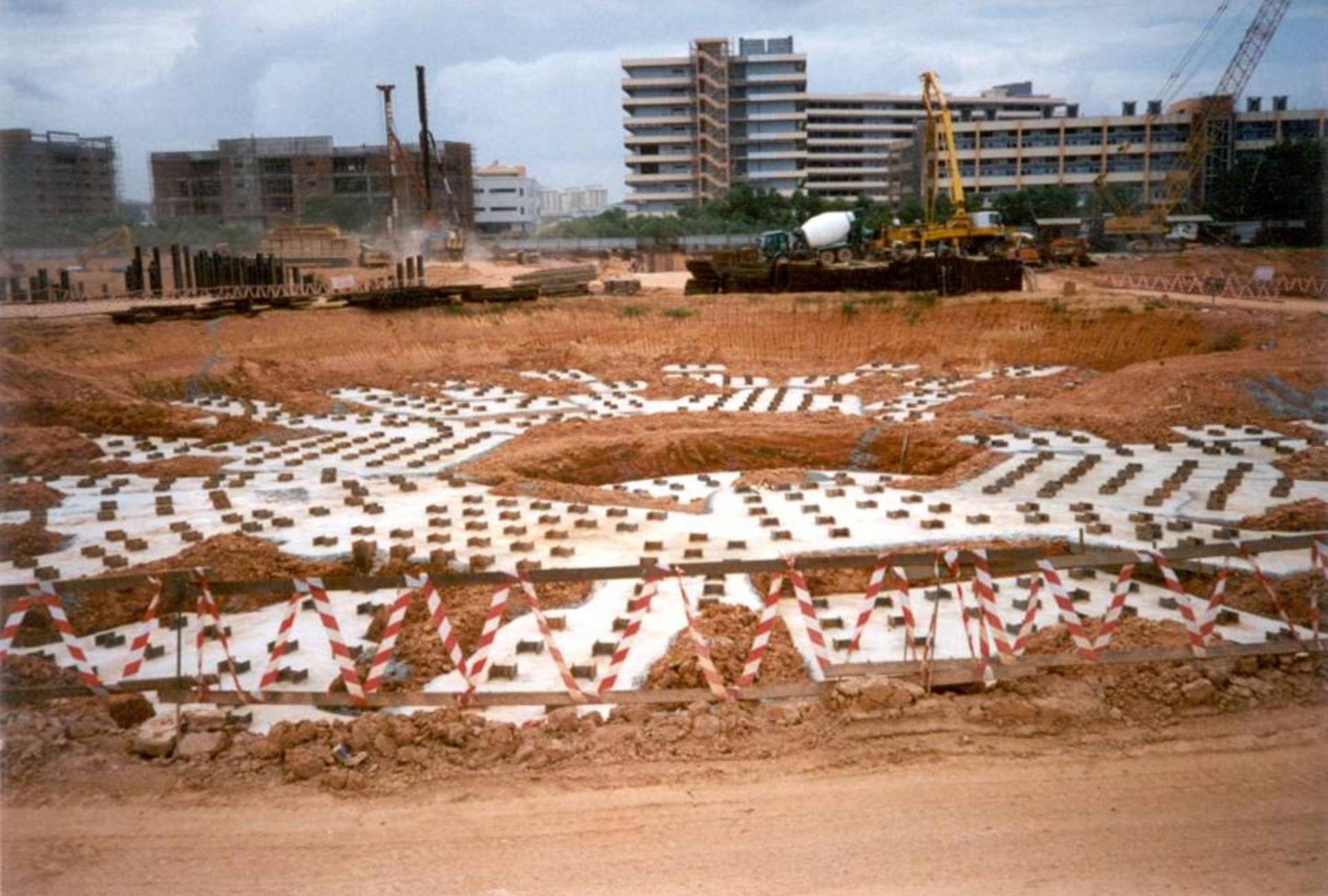
H-Beams for oil storage tanks
