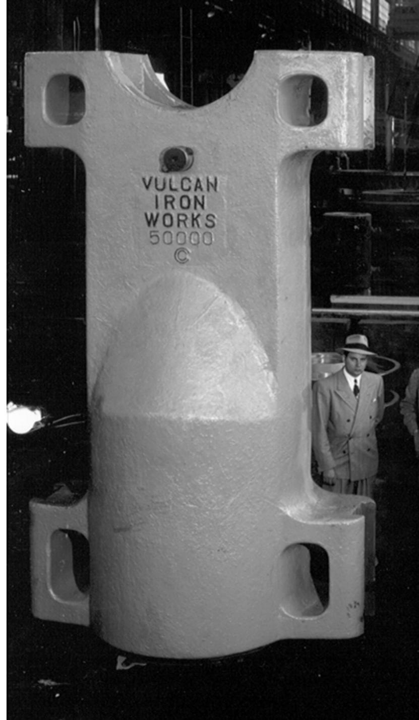
The available impact energy delivered per blow by a drop hammer is calculated simply by multiplying the weight of the hammer times its height of fall.
