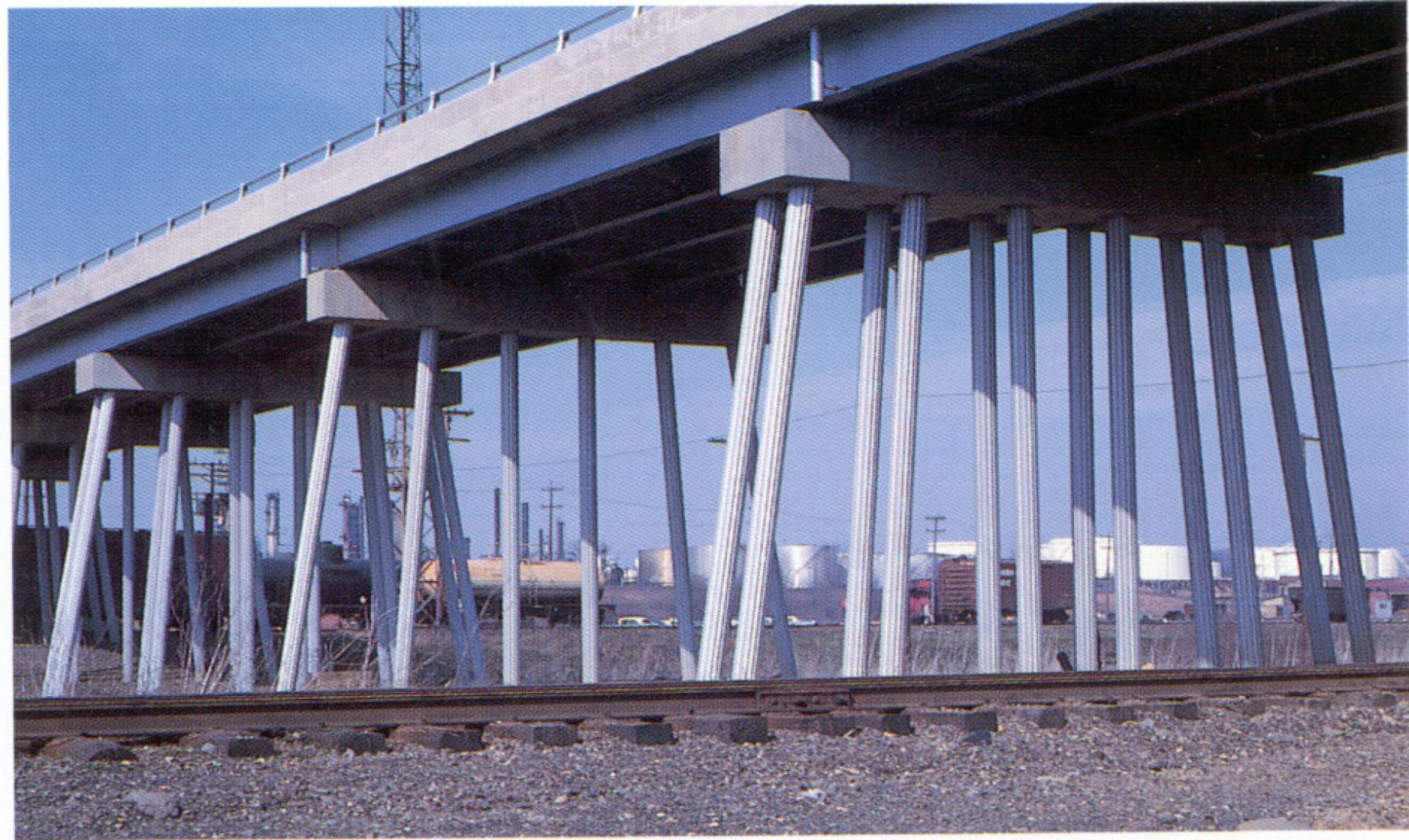
*Monotube piles can simplify design and greatly reduce construction costs when*
