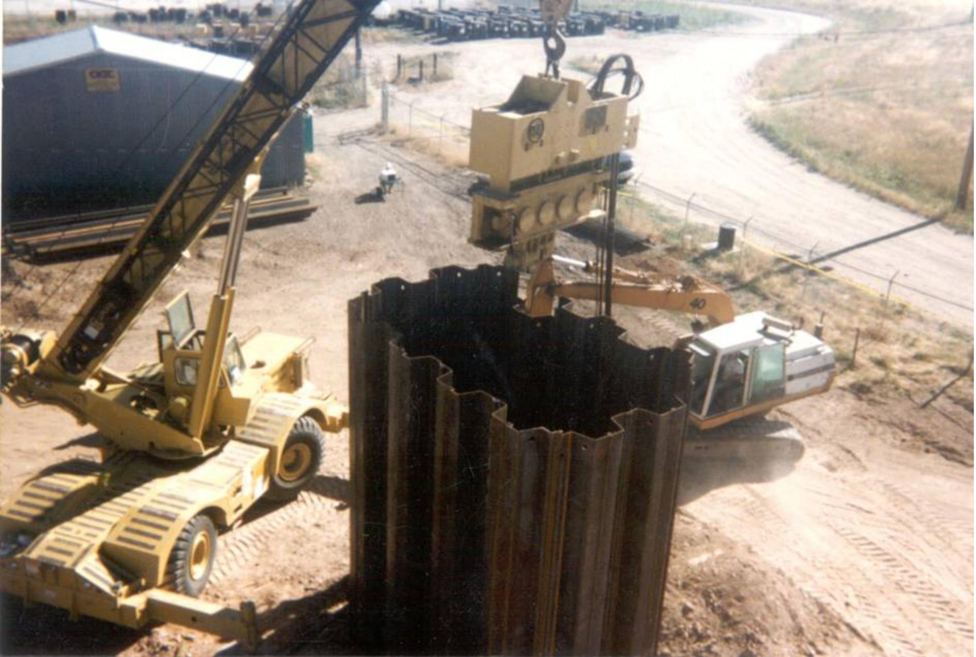
Sheet piles for Air Force missile silos
