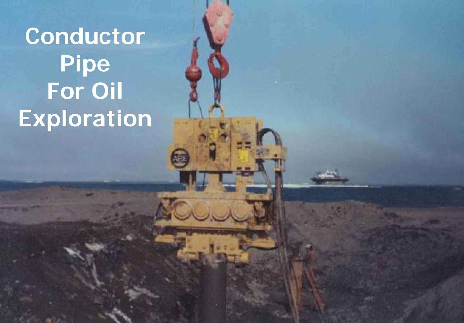
**APE Model 200 extracts 250 foot long conductor pile on North Slope.**
