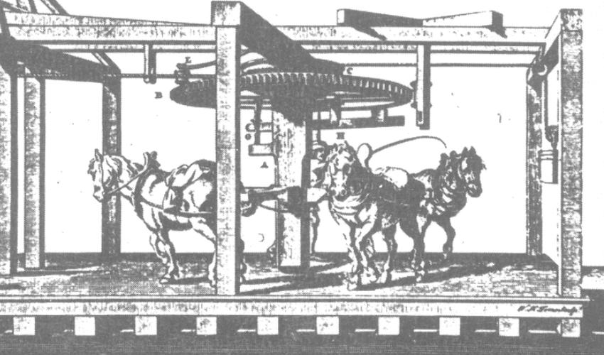
The drop hammer is a heavy weight lifted and dropped on the pile. It operates in guides that position the impact. In the past (and still occasionally) the weight is lifted by man or horse power. Now a line on a crane or a winch raises the weight to a predetermined height where a trip releases it to fall freely on the pile.
